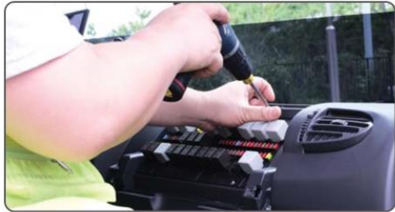
21. Dismantle a fuse box.
